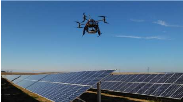
(a) Drone carrying out aerial thermography in photovoltaic plant in Spain
