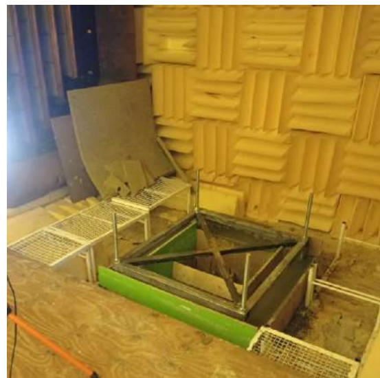
(b) Frame structure installation.
