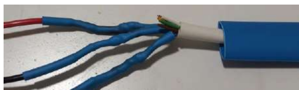
(c) Coating of each individual weld.
