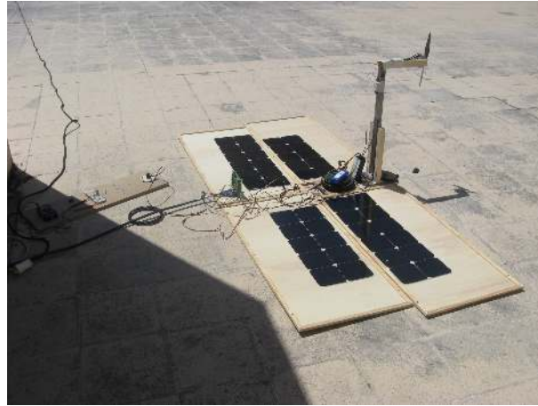
Figure 9.2: Assembly of the full hybrid system used in its testing.
