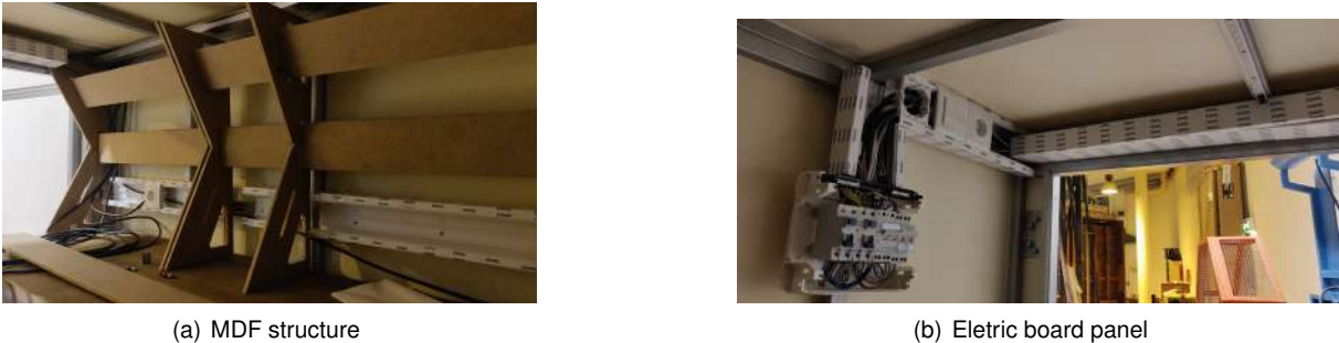
Figure 6.3: MDF structure and electric board panel fixation
